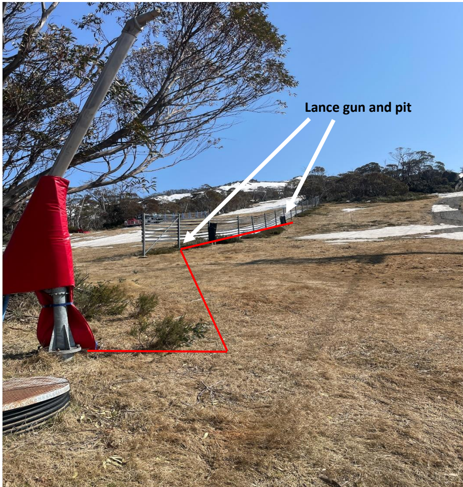
Photo 7: The proposal includes two new lance guns, pits and trenching for power and dialogue cables.
