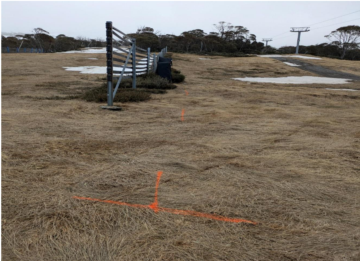
Photo 8: The new lance guns and trenching will result in impacts to the shrubs under the snow fence.
